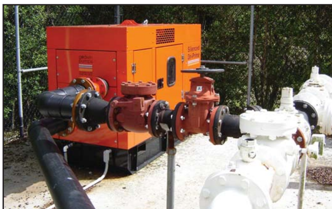
The city of Boynton Beach, FL, purchased this Godwin Dri-Prime Backup System (DBS) unit to provide continuous pumping, particularly throughout the storm season.
